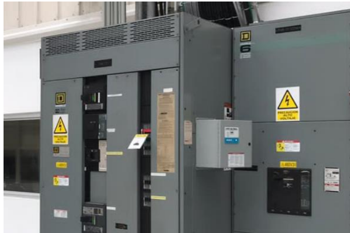
The Surge Protection Devices must be installed close to the service entrance.
