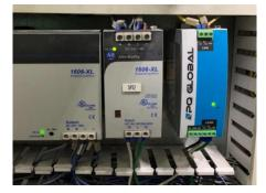
These Surge Protection Devices must be installed close to the critical load
